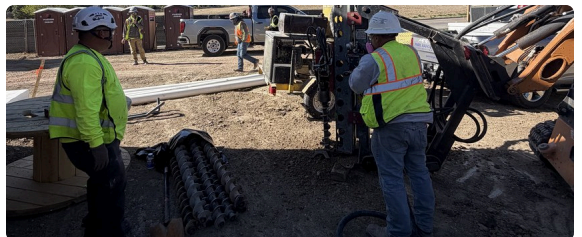
Park Range crew and drill rig on the Erie site.
